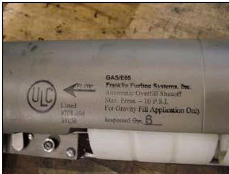
EBW 70849X3Y Autolimiter (Gas/E85 Compatible)
